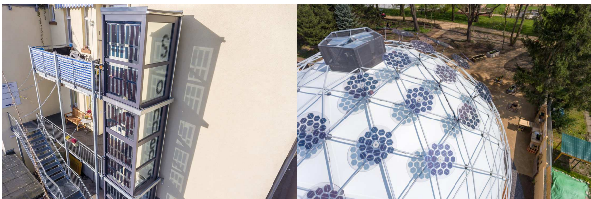
Figure: Glass façade of an external lift shaft comprising organic photovoltaics inlays by OPVIUS (left) and OPVIUS' polycarbonate solar umbrellas on the climate pavilion of the state horticultural show in Thüringen 2017 (right).
